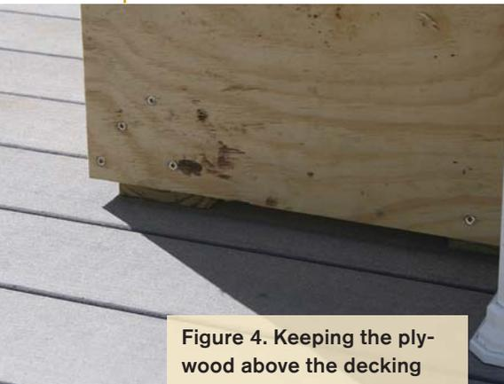
Figure 4. Keeping the plywood above the decking prevents it from wicking water, which could eventually cause delamination.
