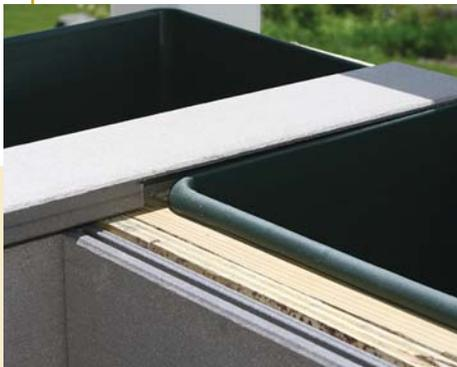
Figure 8. The top of the planter is made from composite decking rabbeted to overlap the liner rims.
