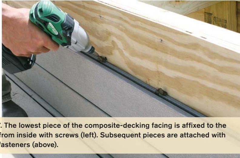
Figure 7. The lowest piece of the composite-decking facing is affixed to the planter from inside with screws (left). Subsequent pieces are attached with hidden fasteners (above).
