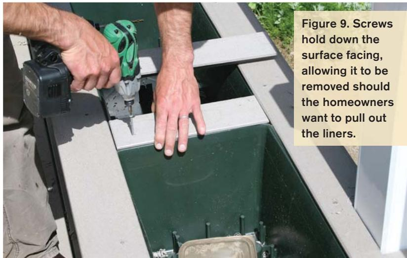
Figure 9. Screws hold down the surface facing, allowing it to be removed should the homeowners want to pull out the liners.
