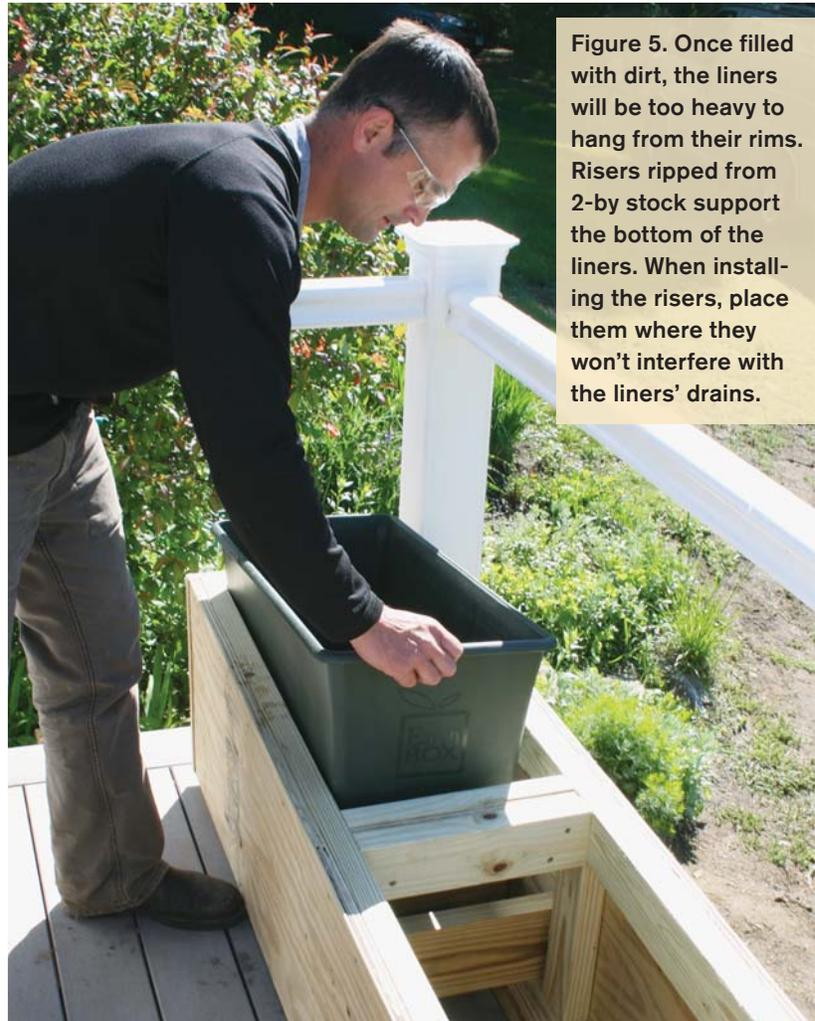
Figure 5. Once filled with dirt, the liners will be too heavy to hang from their rims. Risers ripped from 2-by stock support the bottom of the liners. When installing the risers, place them where they won't interfere with the liners' drains.
