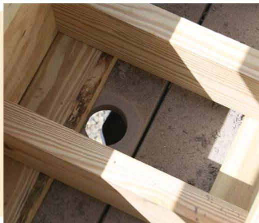
Figure 6. With the liner in place, the author drops a marking pen through its overflow to mark the location of a drain hole (far left). The hole is large — 2½ inches — to prevent clogging (left).
